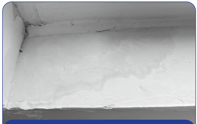
Windowsill Repeated Water Seepage
